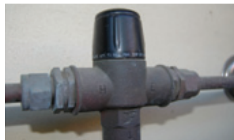
Tempering valves can be identified by either a blue, green, orange or black plastic cap
