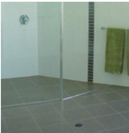
An example of a shower with a level entry
