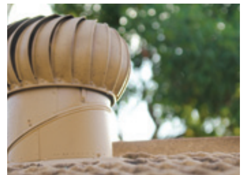
Whirlybirds are a good example of roof ventilation
