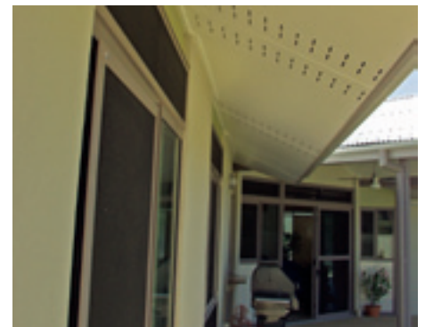
Wide eaves that have vents can reduce heat from the sun by shading windows and help ventilate your home
