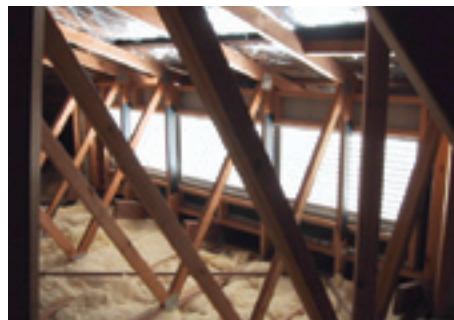
This example shows bulk ceiling insulation and reflective foil on the inside of the roof
