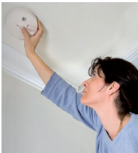
If your home was built before 1 July 1997 it will require at least one 9-volt battery powered smoke alarm
